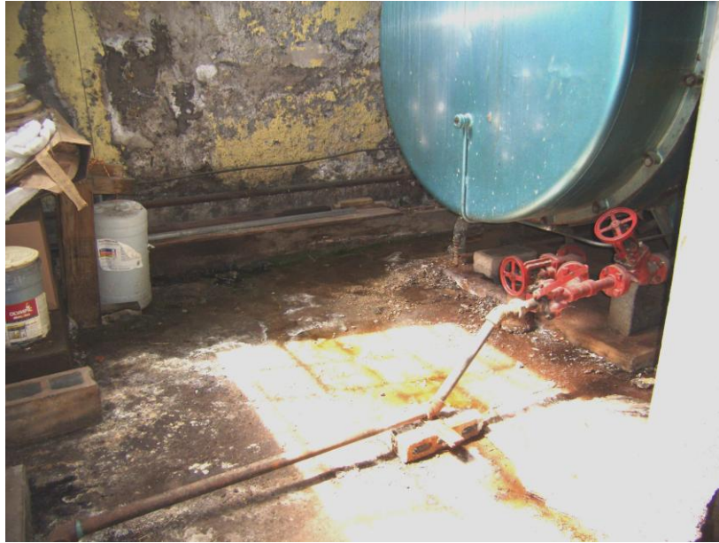
Bio Growth Boiler Room Floor
